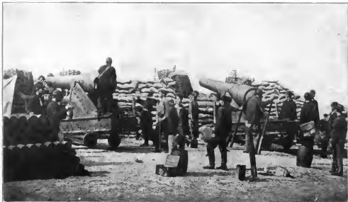
This is a Civil War scene in Battery Meade. The rows of sand bags and the lines of wicker defenses bear a striking resemblance to the methods of fortification that are being used by the soldiers in the modern battery shown below
